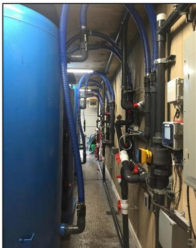
Figure 2. Inside the granular activated carbon treatment system at SANGB
